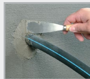
Skim coat with fast-curing cement
