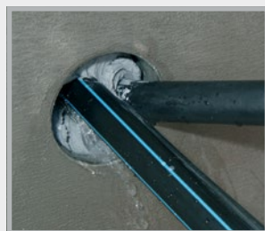
Filling of the annular gap
