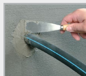
Skim coat with fast-curing cement
