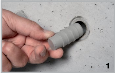
The STOPPER in is pushed into the distance tube.
