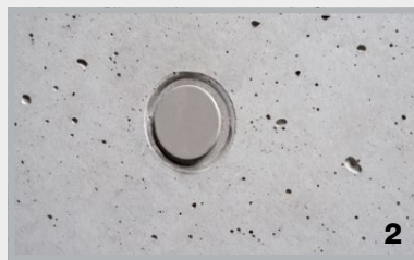
Sealing of distance tube with lip
