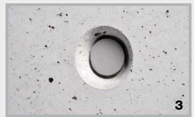
Sealing of distance tube with cone
