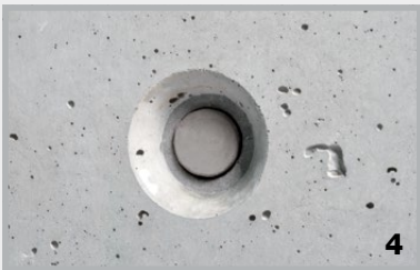
Flush seal for distance tubes with cone.
