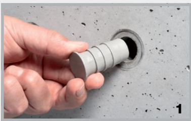
Position and drive in the STOPPER mini
