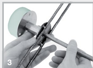
3 Screw axis through the fixing spider and fasten fixed earthing terminal
