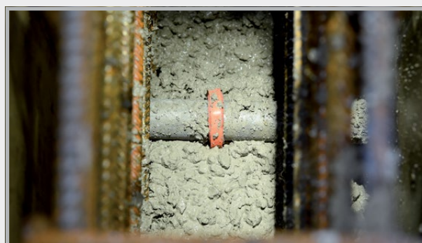
At the construction site
