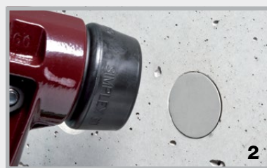
Drive in with rubber mallet
