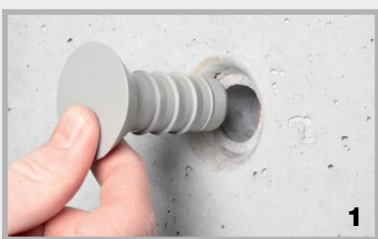
Push the STOPPER maxi into the distance tube
