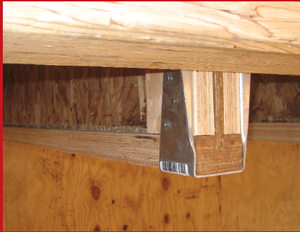
Factory-attached web stiffeners.
