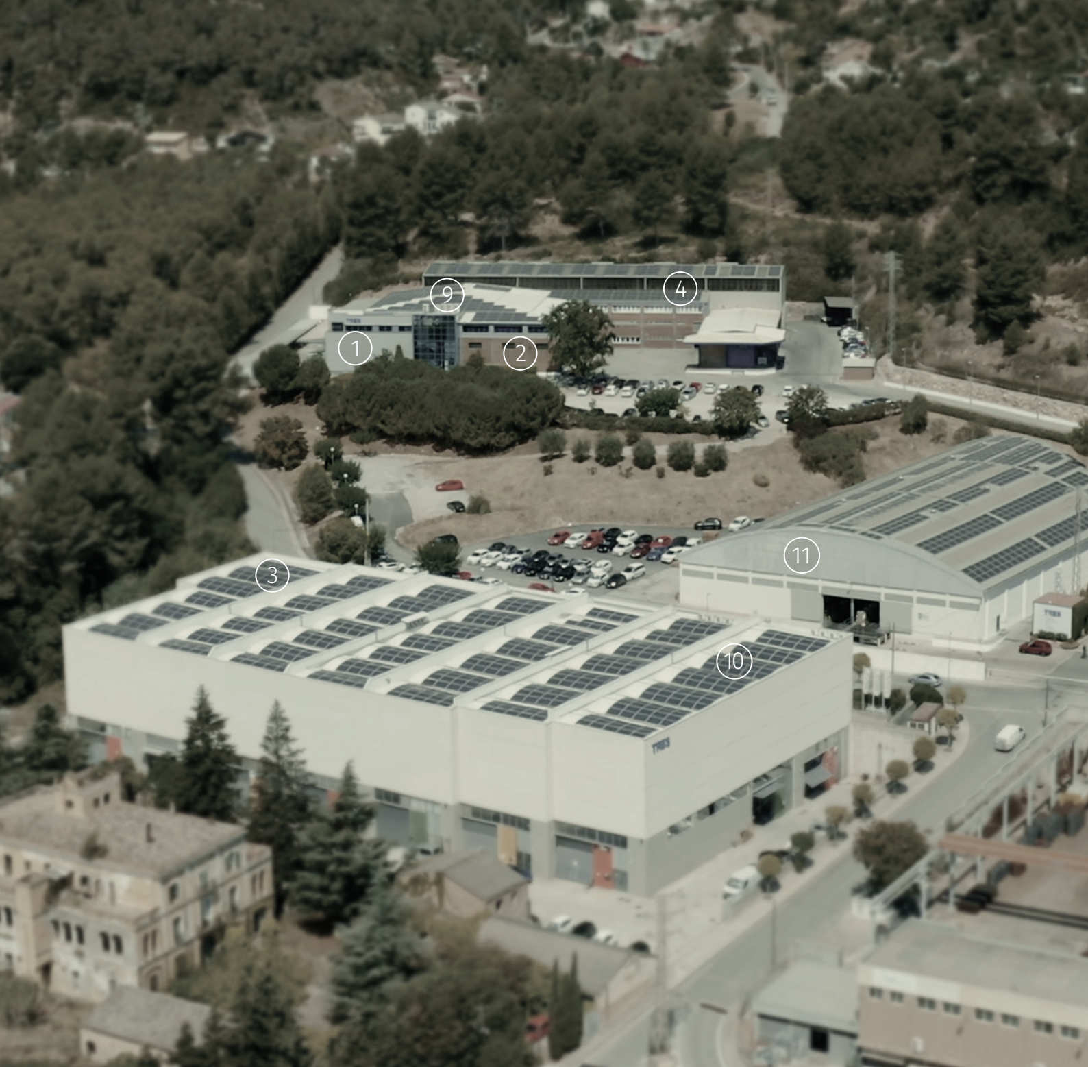
Tres facilities in Vallirana (Barcelona)
